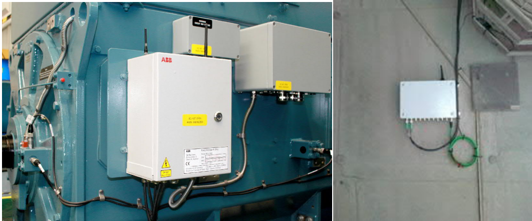
Examples of Mounting DAU on a Machine
