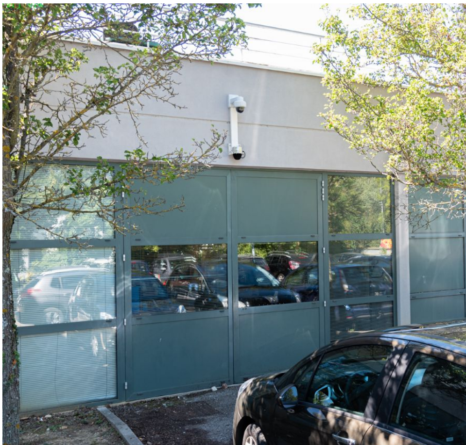
Figure 16: Example of a pod installed on a wall
