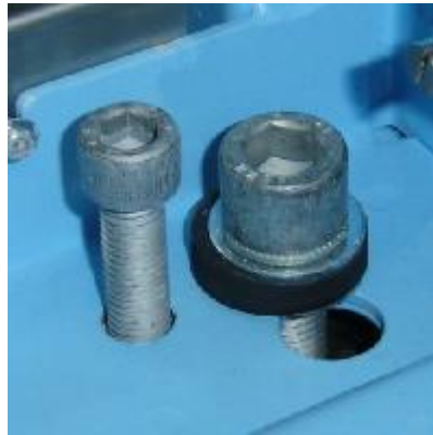
Figure 4: Attachment TVM to Pedestal upon completion
