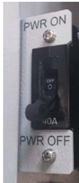
**Figure 3-31 HPR DC Switch**
