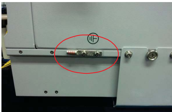
Figure 6-6 Ground Cable Connection (HRU dual side)
