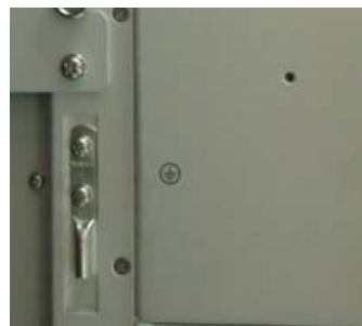
Figure 4-2 Ground Cable Connection
