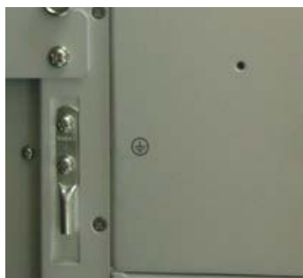
Figure 4-2 Ground Cable Connection
