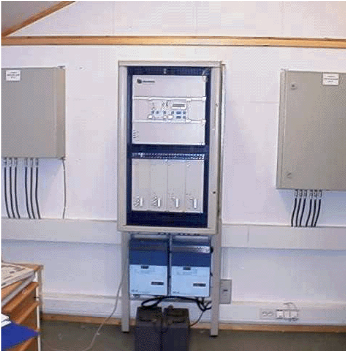
Figure1-4 Glidepath Cabinet Installation
