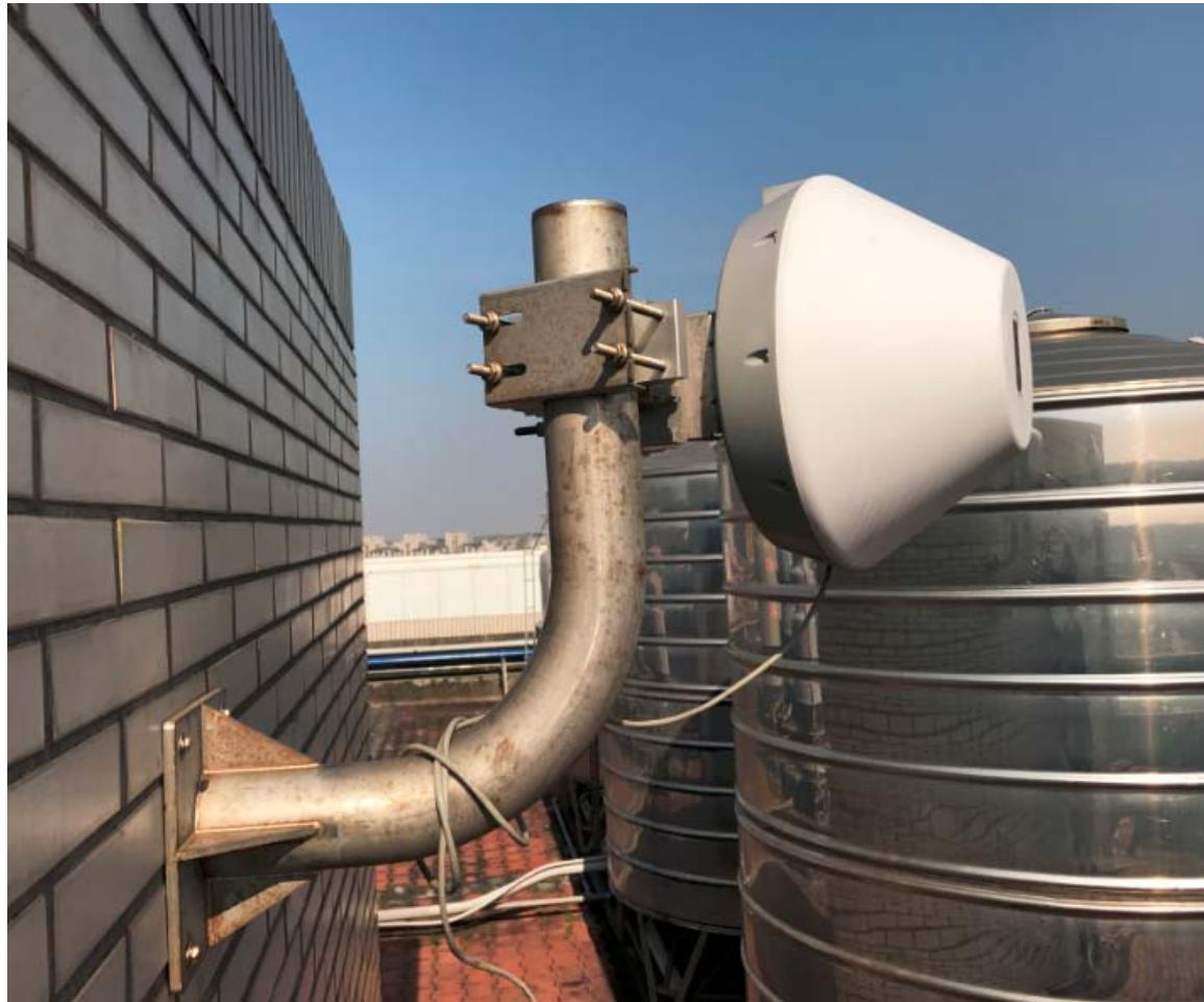
This antenna is normally mounted on a mast and is vertically polarized.
