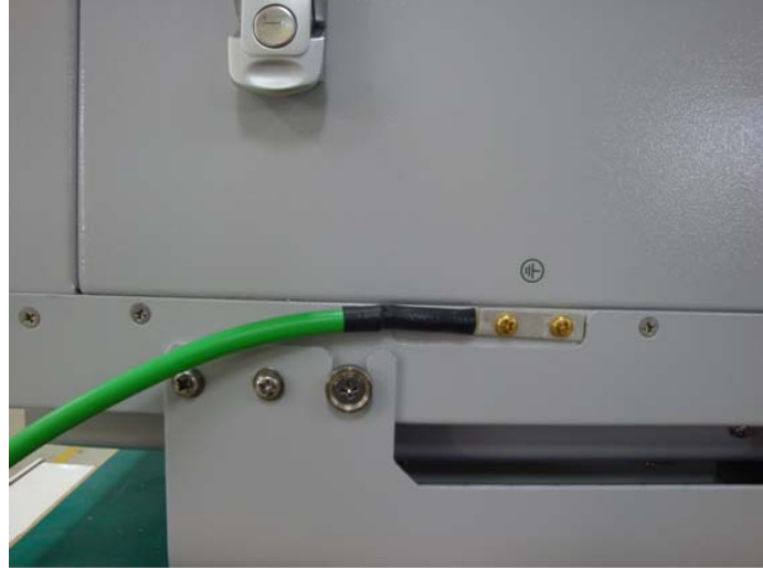
Figure 13 – Ground Cable Connection
