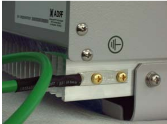
Figure 8 – Ground Cable Connection
