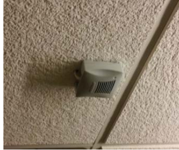
Figure 13: External LF Antenna mounted using the Exciter Mounting Clip
