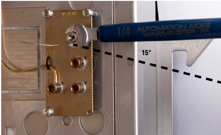
Figure 16 Tightening the connections
