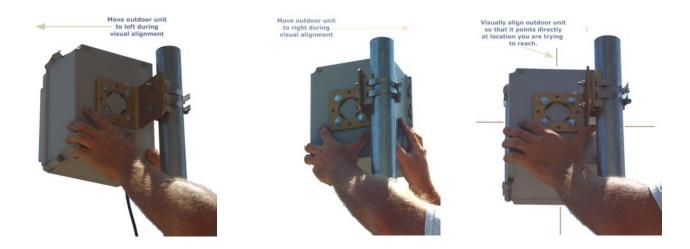
3. Align the external antenna vertically. Loosen the elevation control bolts on the mounting bracket and point the antenna towards the remote end point.
