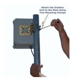
2. Align the external antenna horizontally. Loosen the pole mounting clamps just enough to visually aim the external antenna at the remote end point. Set the appropriate horizontal angle and tighten the pole mounting clamps so that the angle is locked in place.
