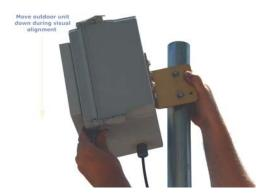
4. Set the appropriate elevation angle and tighten the bolts so that the angle is locked in place. The bracket design allows for up to 20° tilt of the antenna.
