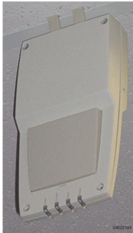
Figure - Clipping the Airespace AP and Ceiling-Mount Clips to a Hanging-Ceiling Rail
