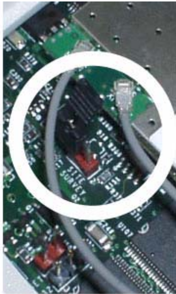
A. Site Survey Jumper Not Installed
