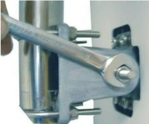
**Figure 19 – HiperMAX-micro SCRT attach SCRT and antenna to pole**
