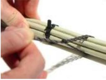
Figure 30 – HiperMAX secure fibre-optic cable, use excess tie
