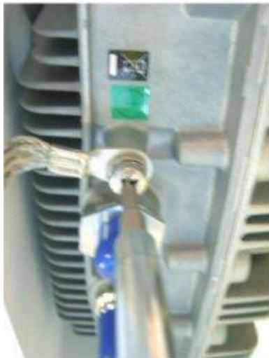
**Figure 21 – HiperMAX-micro SCRT attach earth braid to SCRT**
