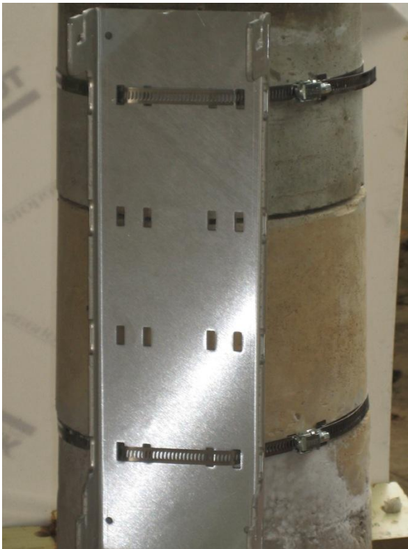
Figure 7 – AirSynergy mounting plate installed (large diameter concrete pole)
