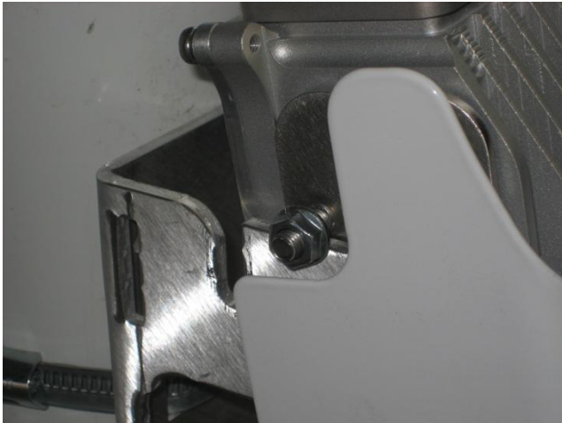
Figure 11 – Lift AirSynergy to top of pole-mount plate
