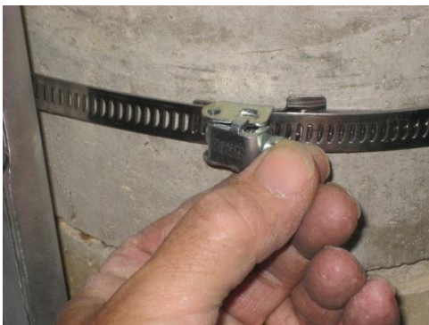
Figure 7 – Press down the locking mechanism with the slack band fed through
