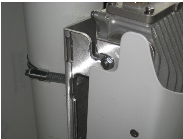
Figure 12 – AirSynergy downtilt adjustment
