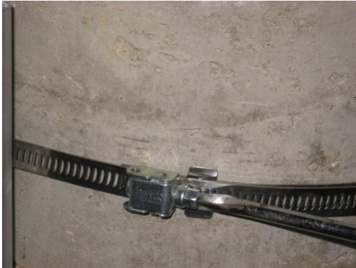
Figure 8 – Tighten clamps with large flat blade screwdriver
