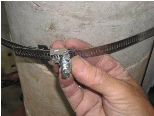
Figure 6 – Feed clamp bands through the quick release locking mechanisms
