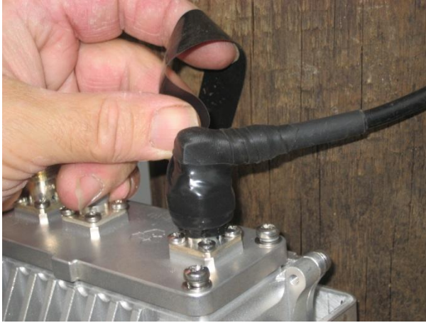
Figure 12 – AirSynergy antenna connections – applying PVC tape
