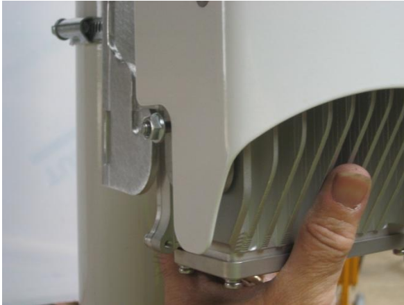
Figure 16 – Gently lift the AirSynergy body until the bottom studs engage in the bottom slots
