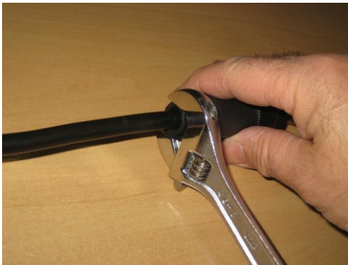
Figure 49 – Assemble the connector and tighten the gland
