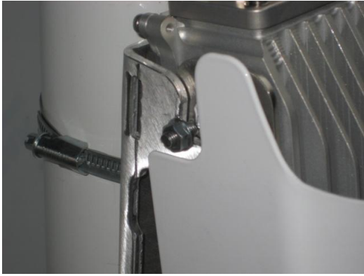
Figure 29 – AirSynergy drops down into slots at the top of pole-mount plate
