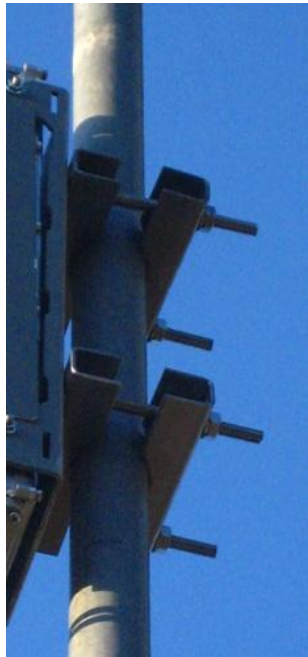
Figure 67 - Mounting method with pole clamps recommended for back to back installations
