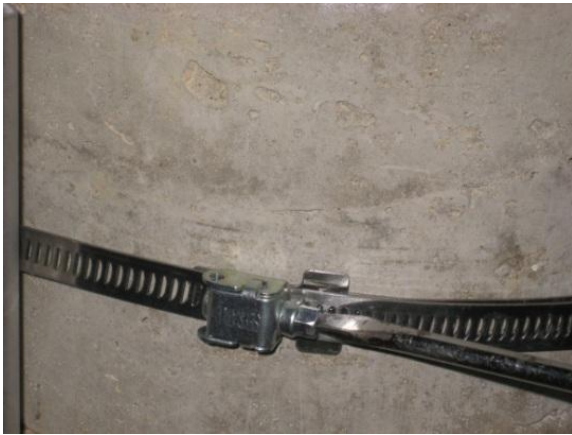
Figure 21 – Tighten clamps with large flat blade screwdriver
