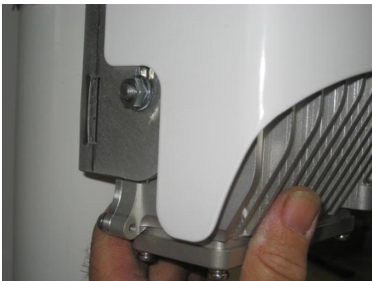
Figure 31 – AirSynergy body engaged in the bottom slots
