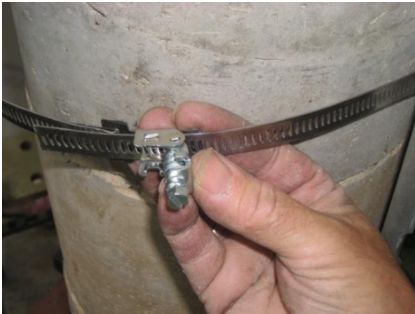
Figure 19 – Feed clamp bands through the quick release locking mechanisms
