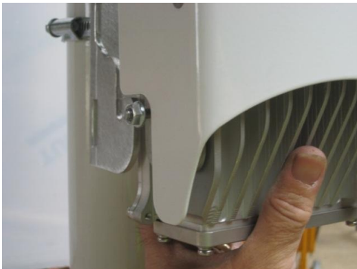
Figure 30 – Gently lift the AirSynergy body until the bottom studs engage in the bottom slots
