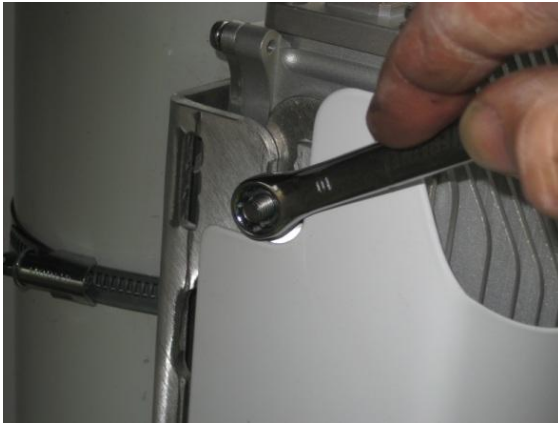
Figure 33 – Tighten flange nuts (4 positions) once the required mounting angle is set
