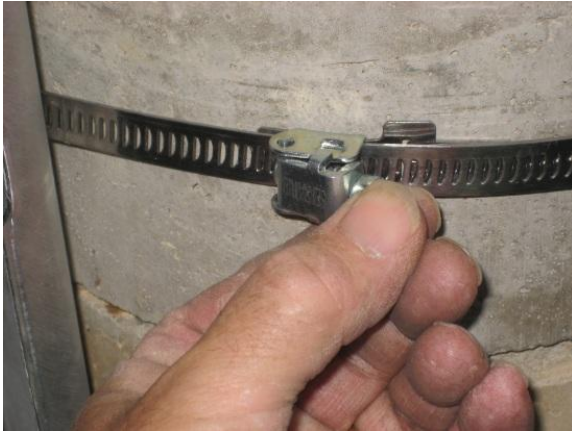
Figure 20 – Press down the locking mechanism with the slack band fed through
