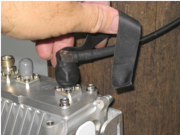
Figure 37 – AirSynergy Front mount antenna connections – applying self -amalgamating tape
