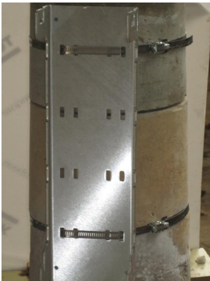
Figure 22 – AirSynergy mounting plate installed (large diameter concrete pole)
