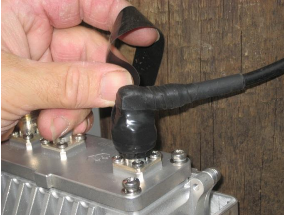
Figure 38 – AirSynergy antenna connections – applying PVC tape
