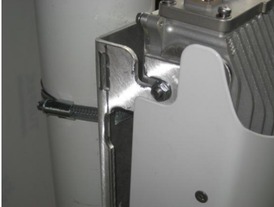
Figure 32 – AirSynergy downtilt adjustment
