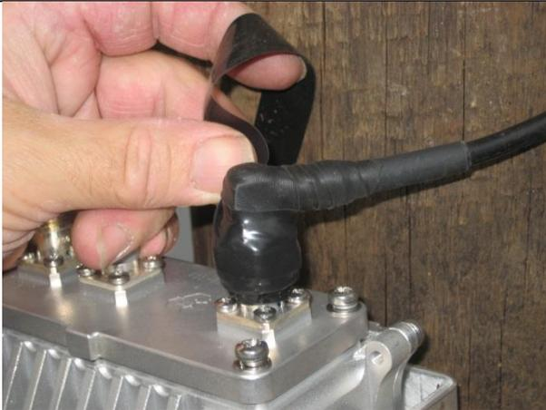
**Figure 35 – AirSynergy antenna connections – applying PVC tape**
