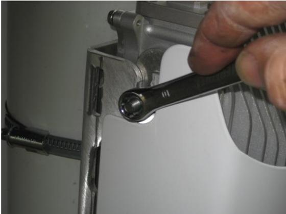
**Figure 30 – Tighten flange nuts (4 positions) once the required mounting angle is set**
