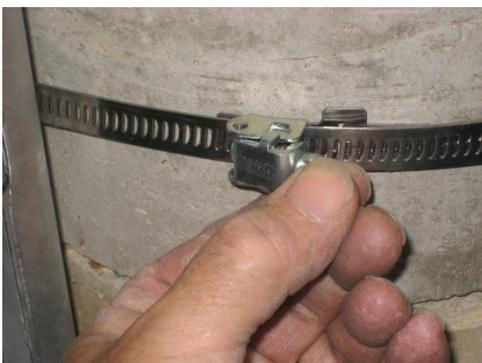
Figure 17 – Press down the locking mechanism with the slack band fed through
