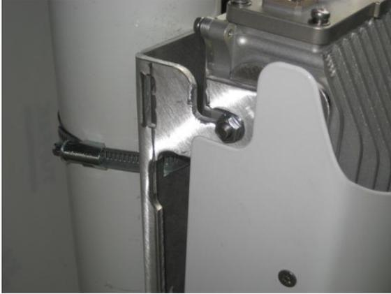
**Figure 29 – AirSynergy downtilt adjustment**
