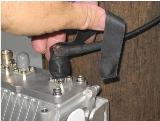
Figure 34 – AirSynergy Front mount antenna connections – applying self -amalgamating tape
