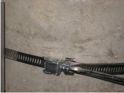
Figure 18 – Tighten clamps with large flat blade screwdriver
