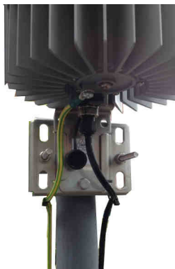
Figure 25: iR460 with Earth and Ethernet Cables Installed
