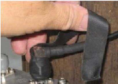
2. Weather-proofing of the RF N type connections is recommended. This is done with a layer of self-amalgamating tape followed by an over layer of PVC tape.
