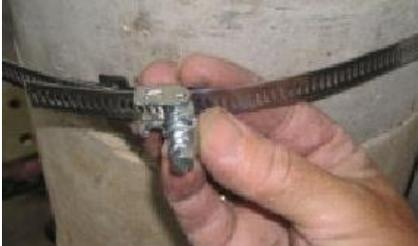
4. Wrap the band to properly fit on the pole. Press down locking mechanism with band excess fed through the mechanism.
