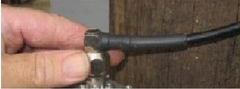
**Caution:** Do not over-tighten the RF connector. RF failures can result when the RF connector is over-tightened.
