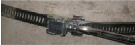
6. Mounting bracket is installed and ready for AC/DC Converter mounting.
