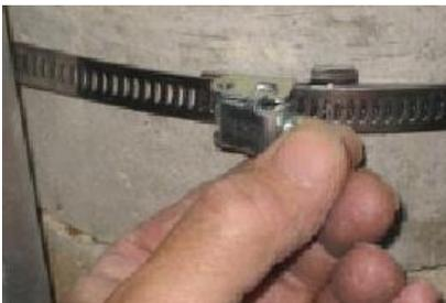
5. Align and position each of the 2 clamps. Tighten the clamp bands with large flat screwdriver in place.
