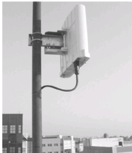
Figure 6-7: Pole-mounted BSR
