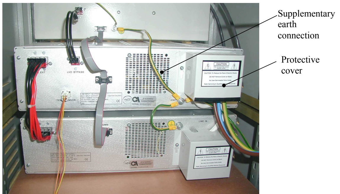
Figure 7-15: Fitting protective covers over terminal block
