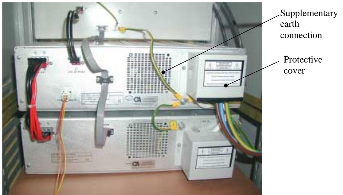
Figure 7-15: Fitting protective covers over terminal block
