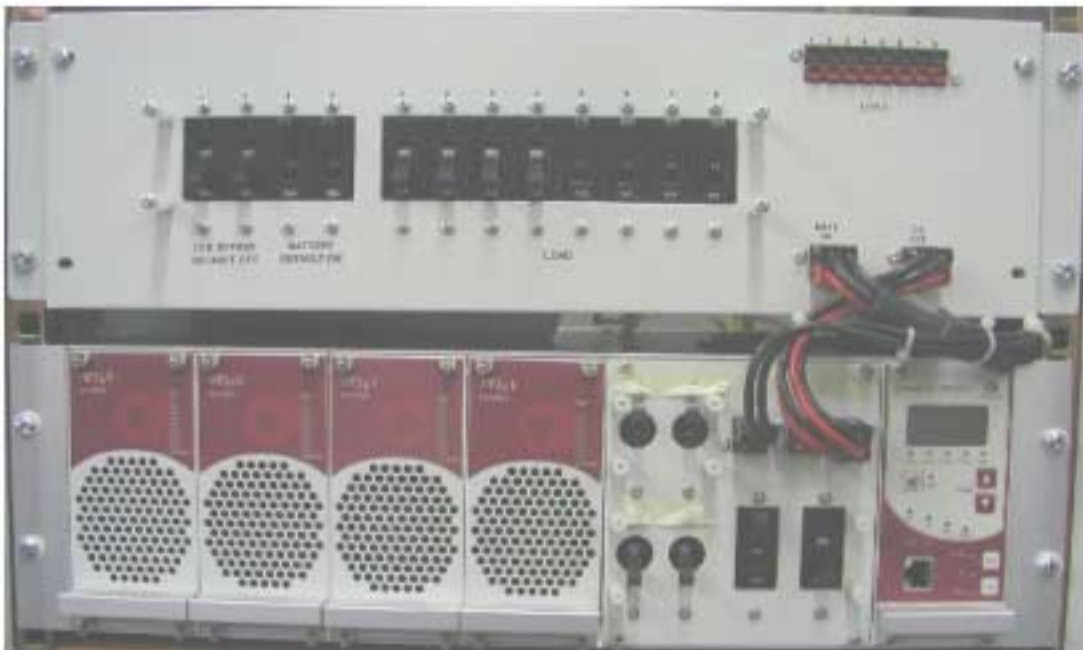
Figure 7-1: BSPS front panel
