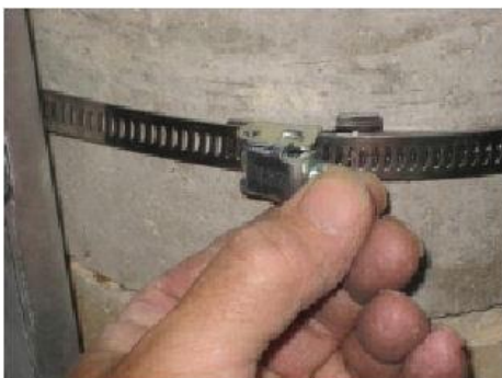
Figure 12: Press down locking mechanism
