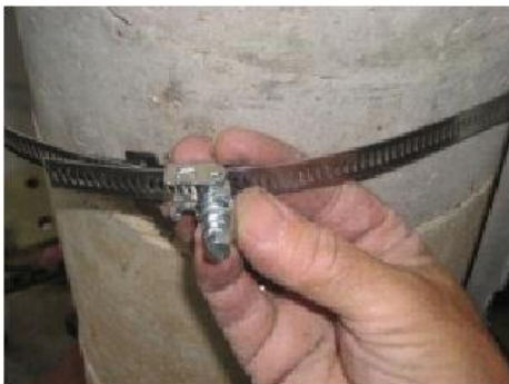
Figure 11: Assemble clamp bands (4 required)
