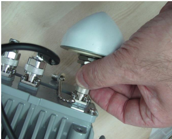
Figure 6: Attaching GPS antenna to unit
