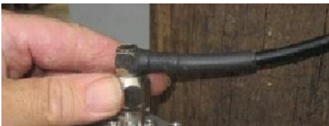
Figure 32: Connecting RF cable
