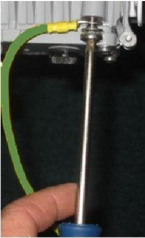
Figure 21: Attaching ground cable to AirHarmony-1000D
