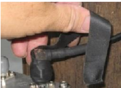
Figure 8: Weather-proof the connection
