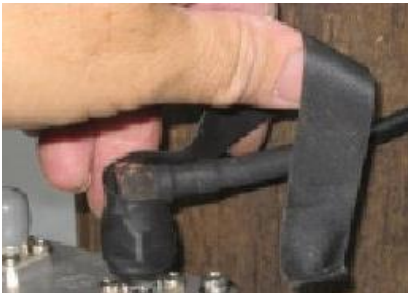
Figure 33: Weather-proof the connection
