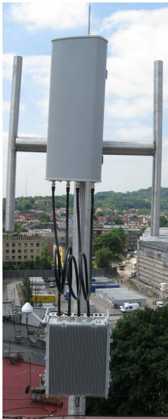
Figure 22 - GPS alternative assembly
