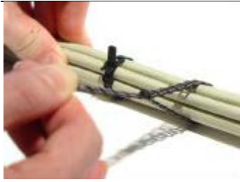
Figure 65 – Secure fiber-optic cable, use excess tie
