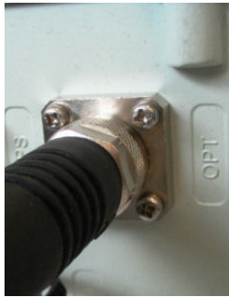
Figure 71 - Fiber-optic cable connected
