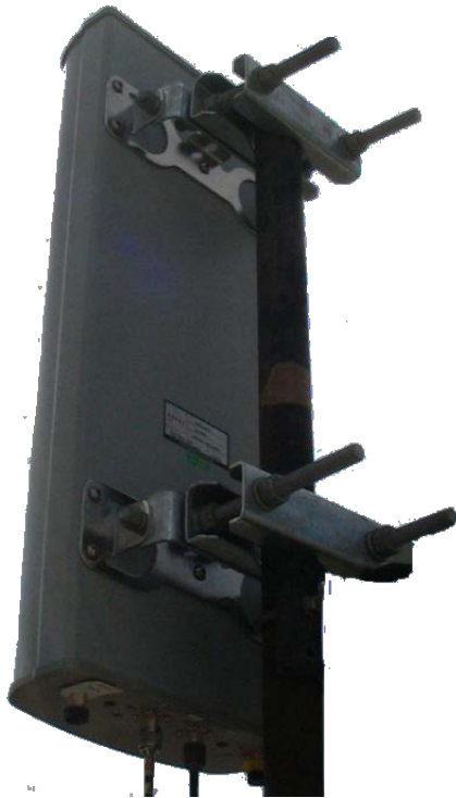
Figure 30 – Air4G Antenna Quad Slant Mast Mount Configuration
