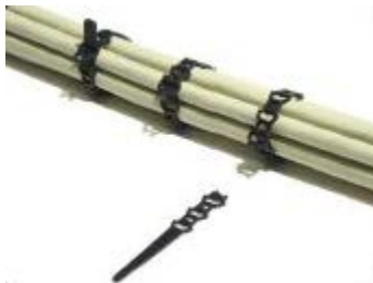
Figure 66 – Secure fiber-optic cable, re-use excess tie
