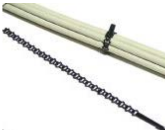
Figure 64 – Secure fiber-optic cable, cut excess tie
