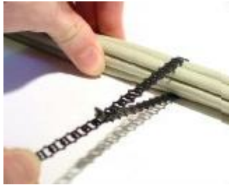
Figure 51 – Secure fiber-optic cable, pull tie
