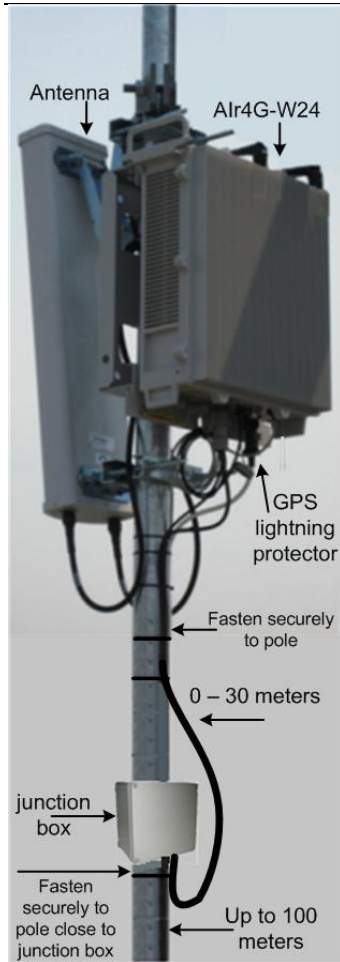
Figure 41 - Air4G-W24 assembly with optional junction box
