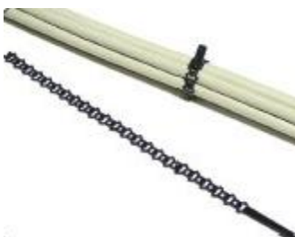
Figure 36 – Secure fiber-optic cable, cut excess tie
