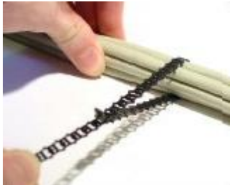
Figure 34 – Secure fiber-optic cable, pull tie
