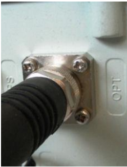
Figure 43 - Fiber-optic cable connected
