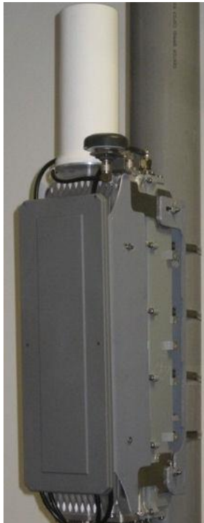
Figure 62 - back to back mounted with 4 straps
