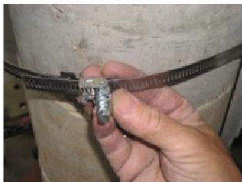
Figure 14 - Assemble clamp bands (2 required)
