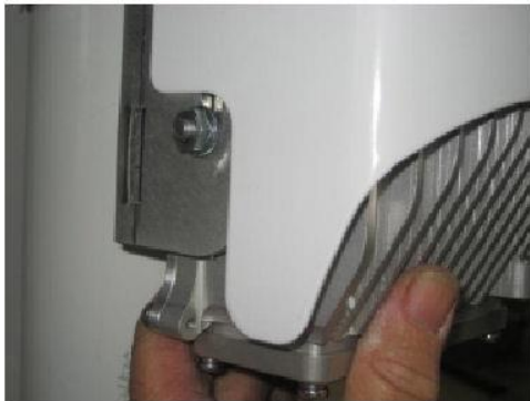
Figure 26 - AirSynergy unit engaged into the bottom slots
