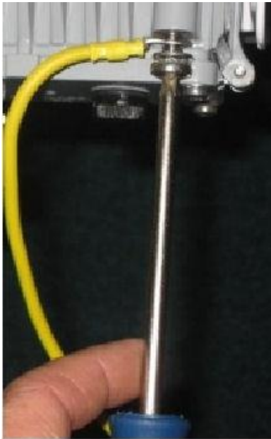
Figure 27 – attaching ground cable to AirSynergy
