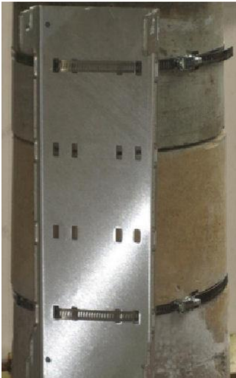
Figure 17 – mounting plate installed on large diameter pole
