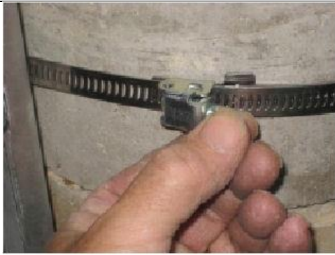
Figure 15 – press down locking mechanism
