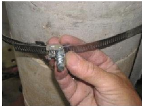
Figure 11 - Assemble clamp bands (2 required)
