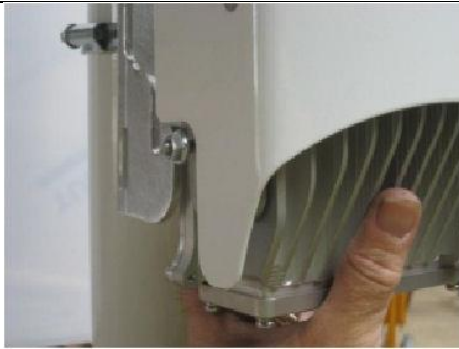
Figure 23 - lift the unit until the bottom studs fit into the bottom slots
