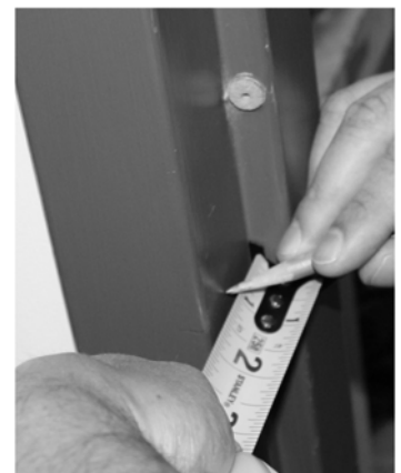
FIG. 12D: LOCATE MAGNET IN JAMB CENTERED DIRECTLY OPPOSITE THE SENSOR WHEN DOOR IS CLOSED
