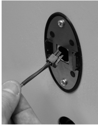
FIG. 7B: FEED THE WIRE INTO THE 5/8" DIAMETER HOLE
