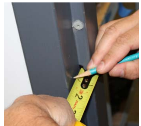
FIG. 6C: LOCATE MAGNET IN JAMB CENTERED DIRECTLY OPPOSITE THE SENSOR WHEN DOOR IS CLOSED
