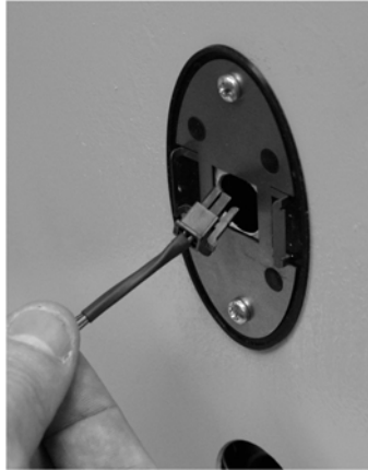
FIG. 14B: FEED THE WIRE INTO THE 5/8" DIAMETER THRU-HOLE (FROM "OUTSIDE" TO "INSIDE")
