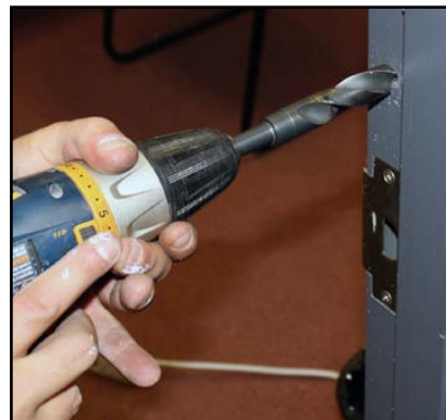
FIG. 10B: DRILL DOOR JAMB HOLE (EITHER 3/8" OR 3/4" DEPENDING ON TYPE)
