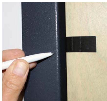
FIG. 6B: CLOSE DOOR AND TRANSFER HEIGHT TO JAMB
