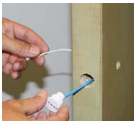
FIG. 13: ROUTE TO THE INSIDE ("PROTECTED") SIDE OF THE DOOR
