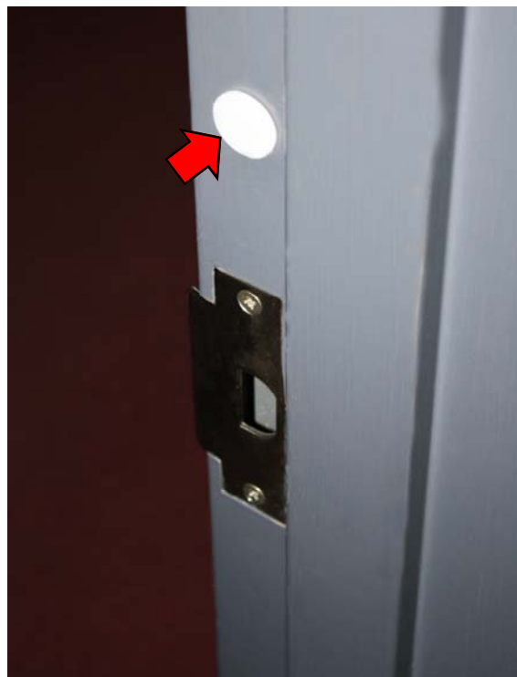
FIG. 10C: DOOR CONTACT MAGNET INSTALLED IN DOOR JAMB
