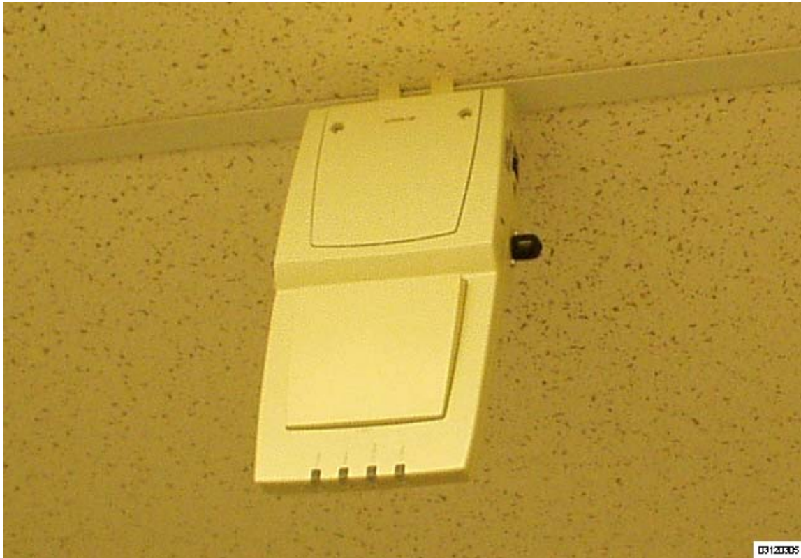
Figure - Clipping the OmniAccess AP and Ceiling-Mount Clips to a Hanging-Ceiling Rail
