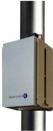
Pole mount installation
