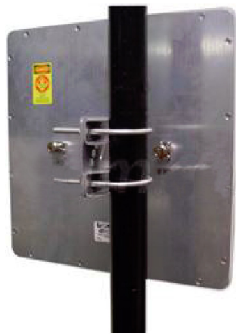
Figure 31. Installing Flat Panel Antenna to the Pole
