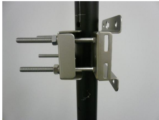
Figure 13 Completion of Mounting
