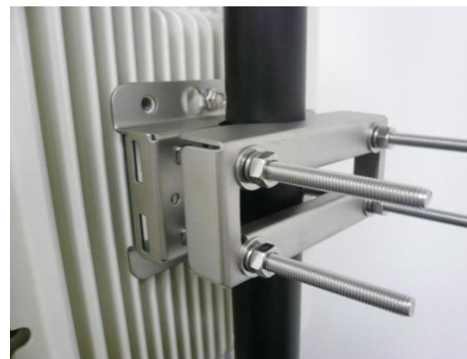
Figure 15 Clamping and secure the unit on pole
