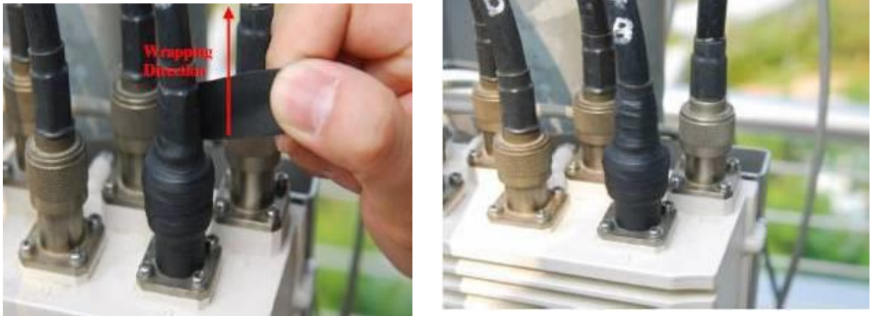
Figure 29. Wrapping direction and extends the wrap 1" above the connector clamping
