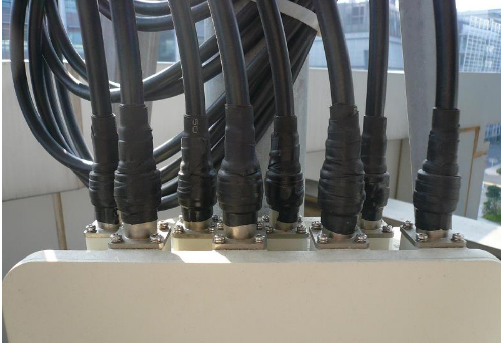
Figure 27. Wrap the Butyl Rubber Strip
