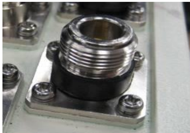
Figure 28. Butyl Rubber Ring Finished
