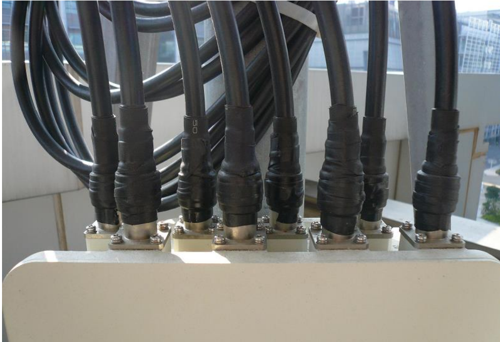
Figure 27. Wrap the Butyl Rubber Strip
