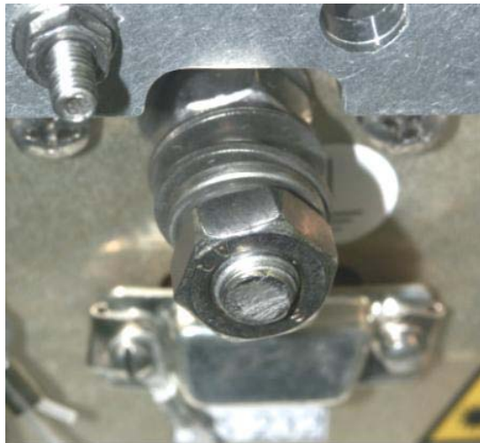
figure 3-7 Grounding bolt with loosened hex nut
