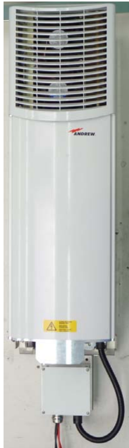
figure 3-8 Mounting of DC Box, finished
