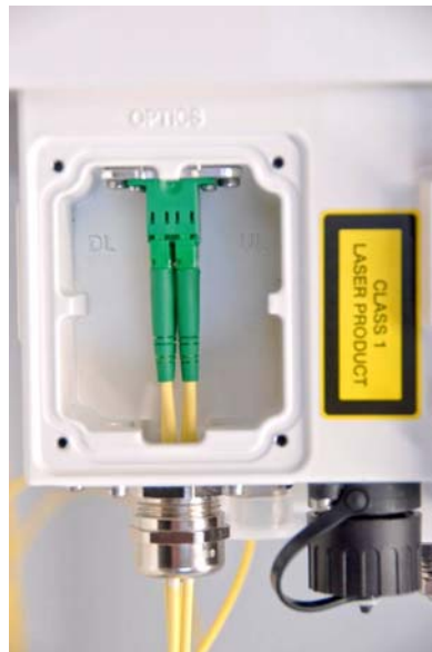
Figure 2-23 Optical cable installed
