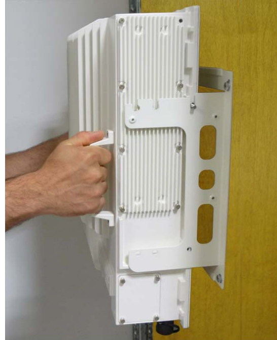
Figure 2-6 Place RU onto wall mounting bracket
