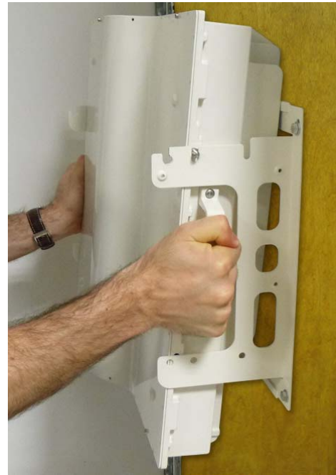
figure 4-10 1 st RU placed on wall mounting bracket - MIMO
