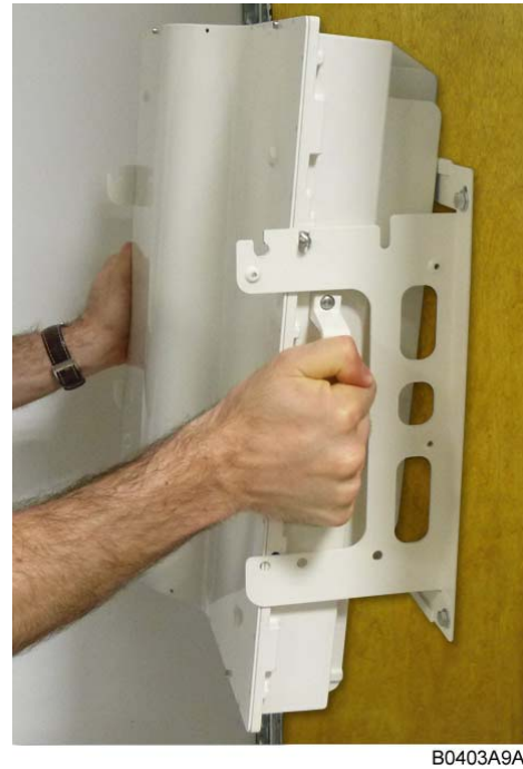
figure 4-10 1 st unit placed on wall mounting bracket
