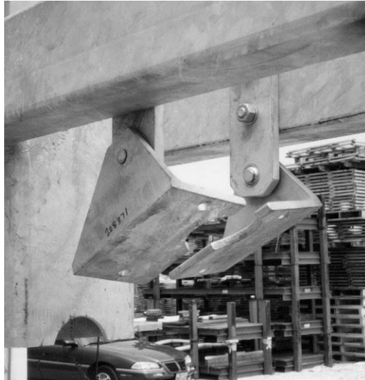
Figure 3-27: Elevation Pivot Bracket Assembly
