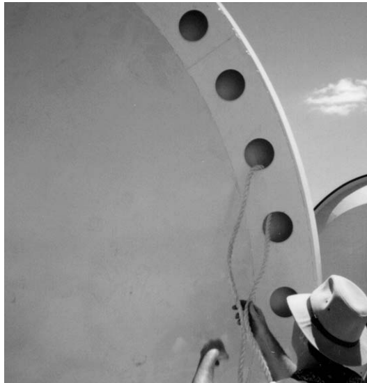
Figure 3-43: Safety Rope Tag Lines
