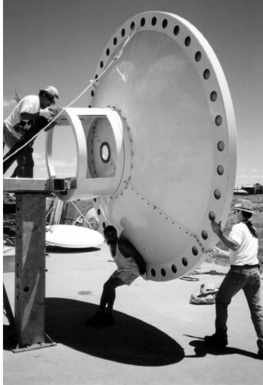
Figure 3-49: Elevation Jack/Enclosure Attachment
