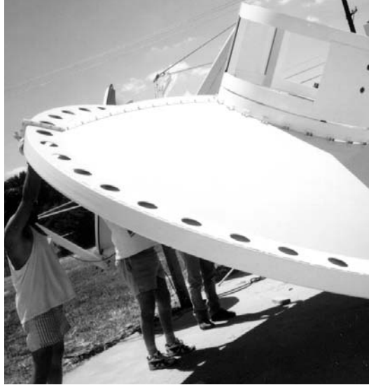
Figure 3-45: Manual Lift of the Reflector to the Mount
