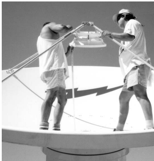
Figure 3-55: Subreflector Alignment
