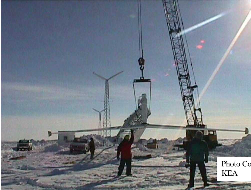
Figure 6-12 Lifting of tilt down tower at Kotzebue Electric Association
