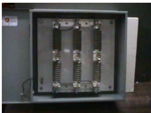
Figure 12.1-3 Dynamic brake resistors
