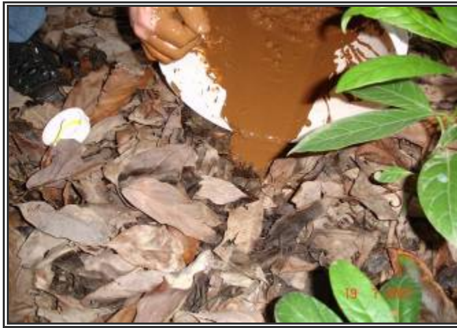
Figure 8: Pouring slurry from the augured hole back into the hole
