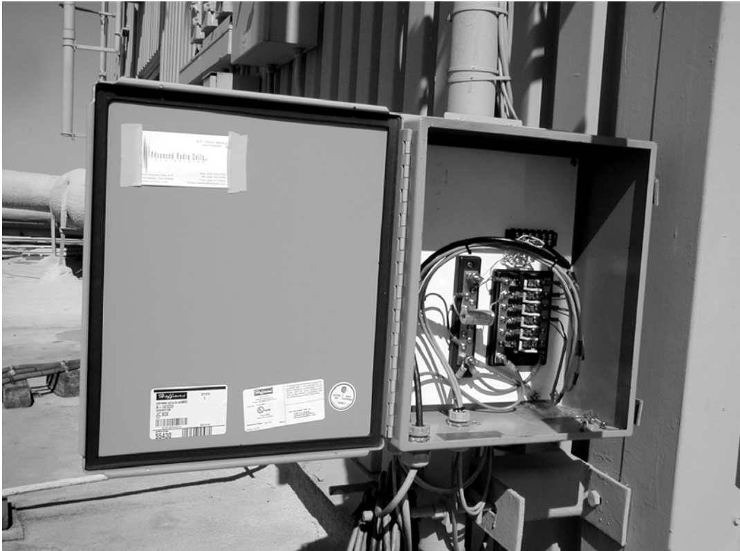
Figure 5-6: Photo of open OJB.
