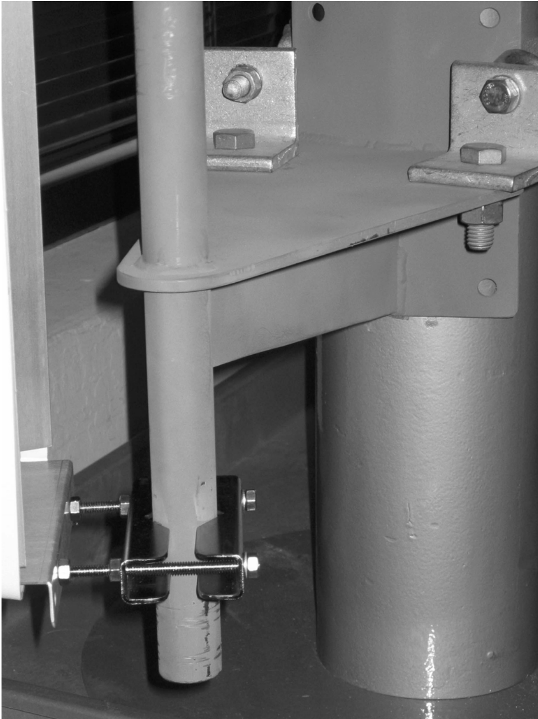
Figure 3-9: Pole Mount Kit and pipe mounted AP detail.
