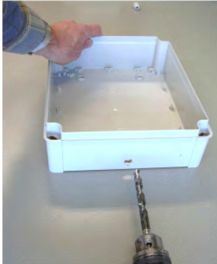
Figure 72: Drilling the hole (12 mm)
