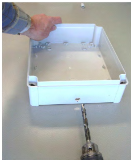
Figure 61: Drilling the hole (12 mm)
